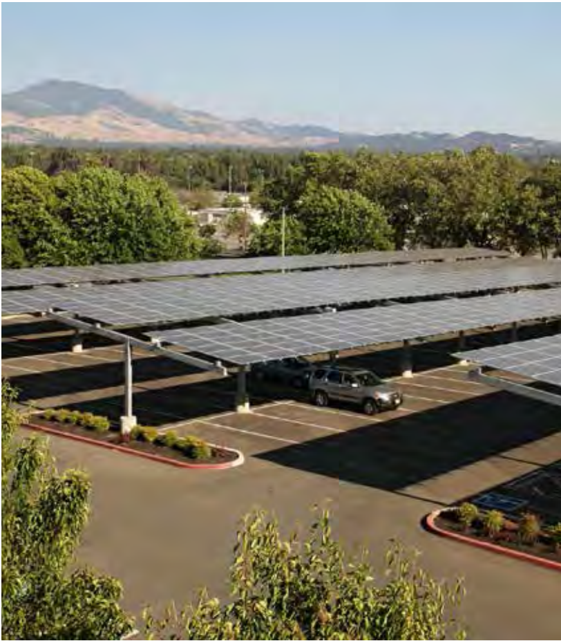
Garage Rooftop solar arrays
